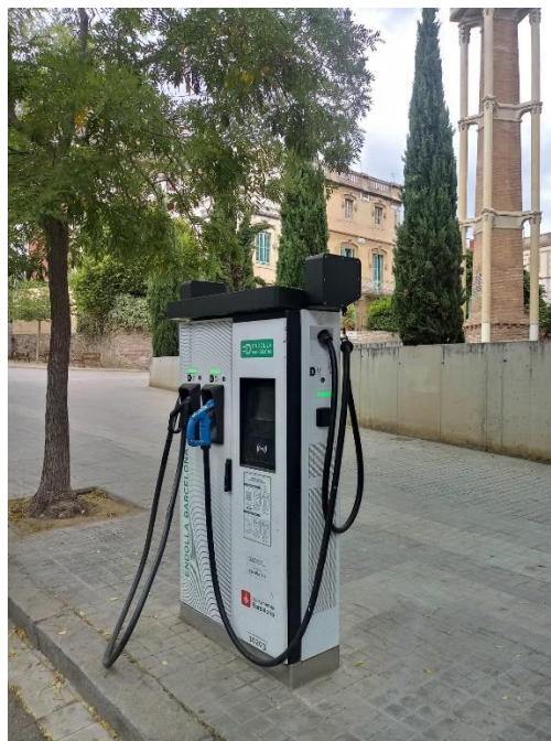
Figure 12. Charging point with a retractable cable with 6m length.
