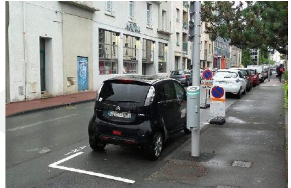
A charging point on lamp post in la-Roche-Sur-Yon
