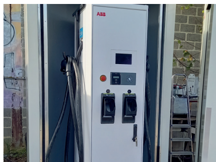
ABB 180 kW Terra charger in mobile container
